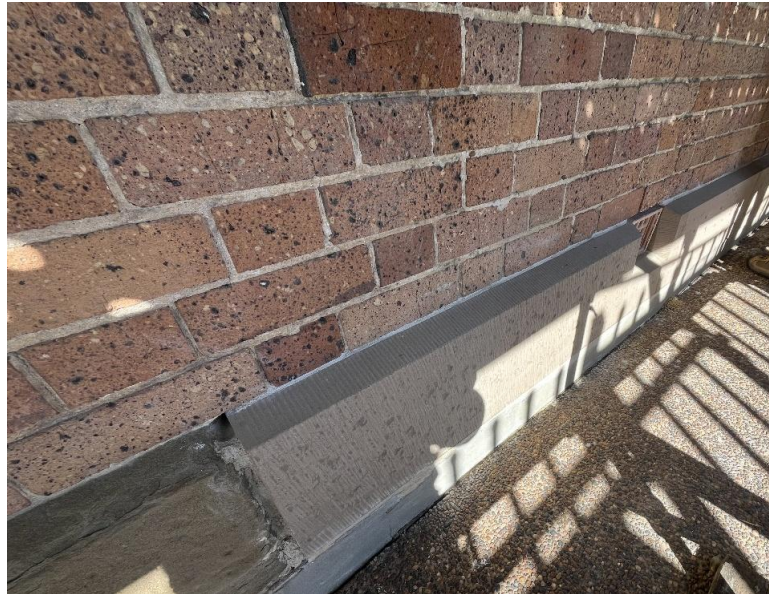
Image above: external features of Building B after façade stonework restoration.
